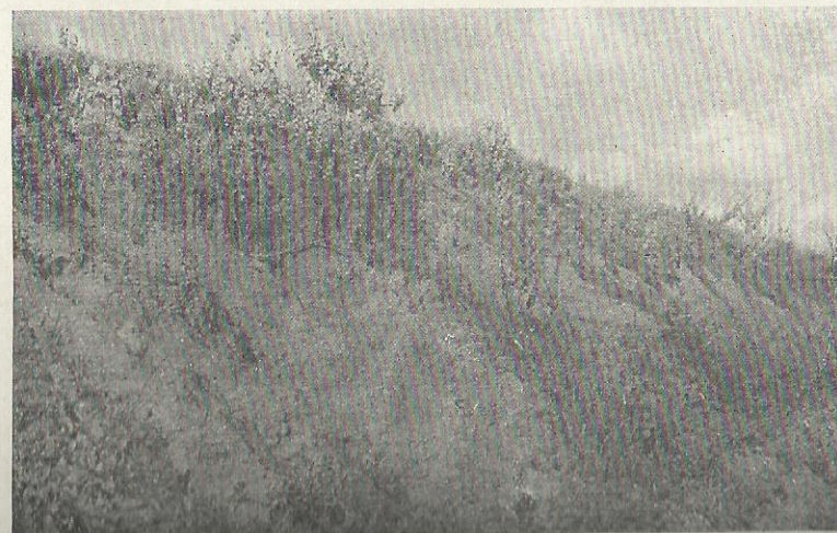
A road-cut at Cullis, Hermosa. The soil is Cullis loam, an erosive soil. Such exposed cuts should be protected by planting them to quick-growing grasses or shrubs.
