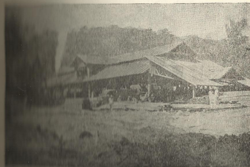
Figure 11. Tapan Lumber Co. at Sanchez-Mira, Cagayan. The daily capacity of this sawmill is about 15,000 board feet.
