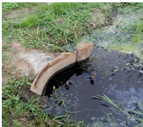
Figure 2.5 Culvert that serves as check gate to control entry of irrigation water/ salt water
